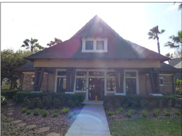
Activity Center Front View
